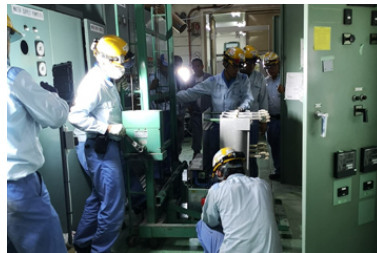
Replacement of equipment
