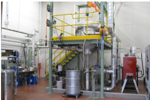
Dissolution plant exterior
